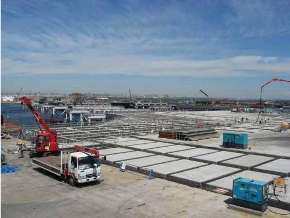
(Photo No.8 Construction Site of Haneda Airport)
