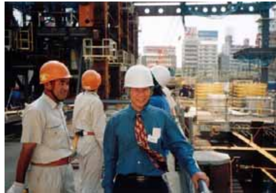
Construction Site in Shinagawa
