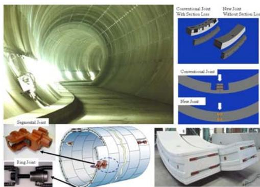
Figure 4 RC Lining Segment with Rigidity Controllable One-Pass Joints
