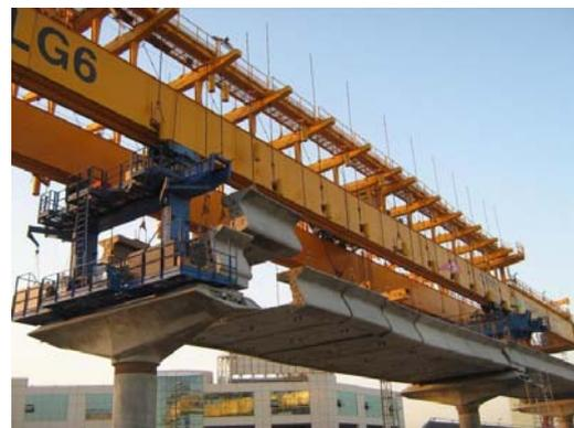
Viaduct Segments erected by a Launching Gantry
