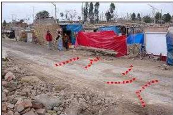
Figure 3. Ground tension cracks in front of collapsed houses
