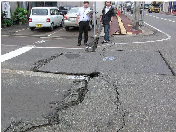
**Photo. 1:** Crack opened along ridge of sand dune
