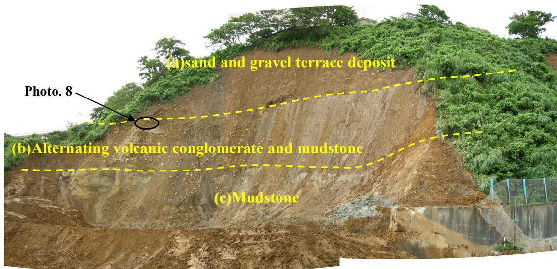
**Photo 7:** Failure surface with geological stratification.
