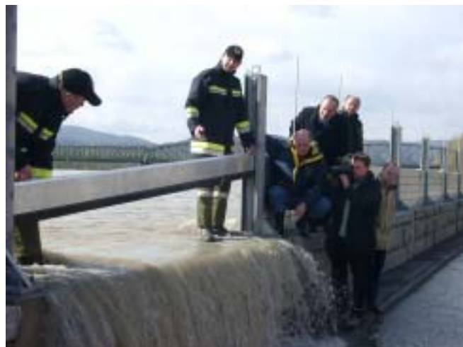
Photo-3 Mobile levees at Krems along Danube River (Courtesy of Municipality of Passau)
