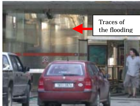
Photo-1 Traces from the flooding at the subway entrance (Prague)
