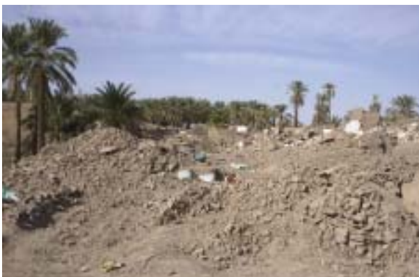
Photo-5: Collapsed adobe structure houses
