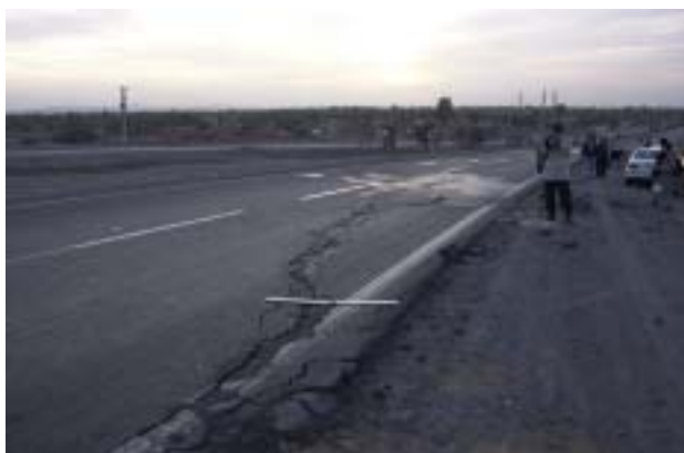
Photo-2: Crack on the road traversing the flexural scarp
