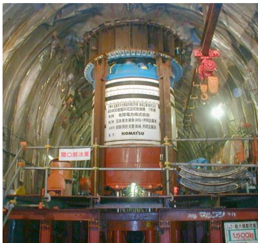
Photo 6 : Excavator for the pilot shaft
