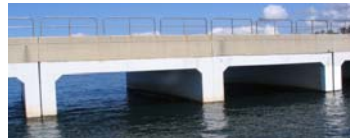
Photo 2 : An abutment with culverts
