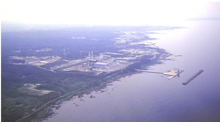
Photo 1 : Panoramic view of Shika Nuclear Power Station
