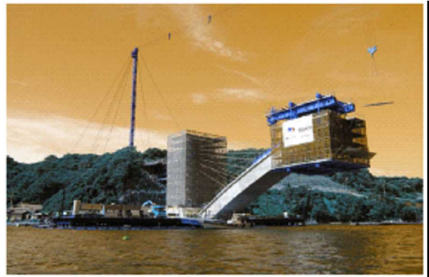
Photo 2 Overhang Construction
