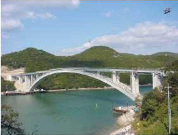
Photo 1 Construction of the Kashirajima Bridge
