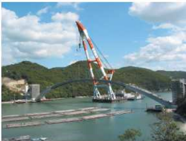
Photo 4 Simultaneous Construction of Melan Material
