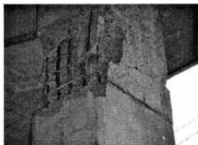
Photo 9 Muramatsu viaduct (fallen concrete)
