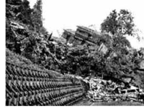
Photo 5 Failure of residential land developed on the talus layer in Nigorizawa
