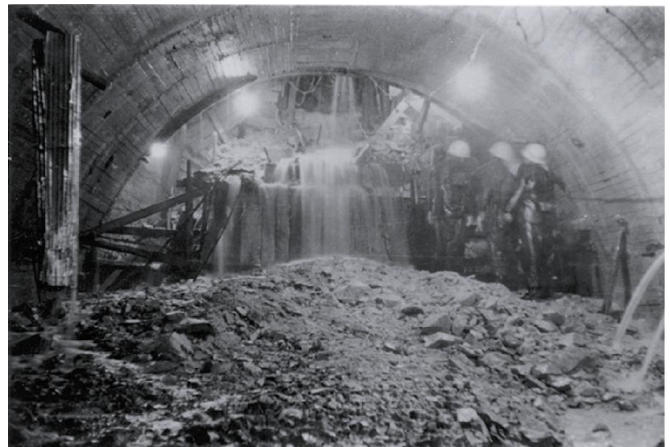
Photo-2: Fractured zone at the heading of the Kanden Tunnel. (1957)
