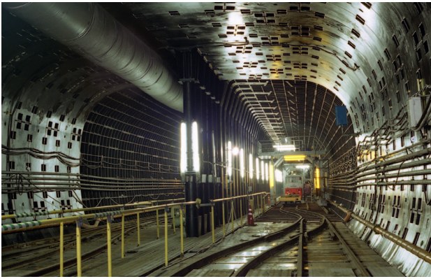
Photo 2: Connecting part of two different sections
