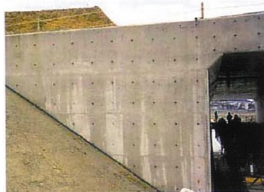
Photo 1: Box culvert prior to the repair
