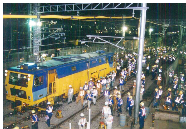
Photo3. Re-routings (utilization of a large-sized track maintenance machine)
