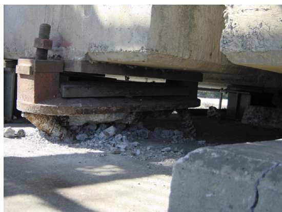
Photo 8: Rekifune Bridge; Loosened anchor bolt
