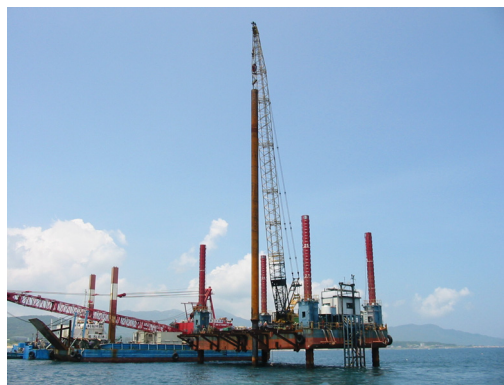
Photo-1: Steel pipe sheet pile driving work by a vibro hammer
