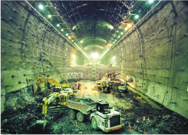
Photo 2: Underground power plant undergoing excavation
