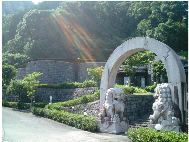
Photo 1: Sekisho-kan: Building made of indigenous welded tuff is suited to pass down the stonemasonry to the future generations.
