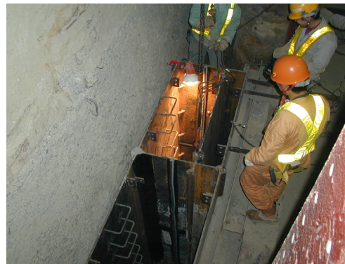
Photo 2: Constructing JES toward Length
