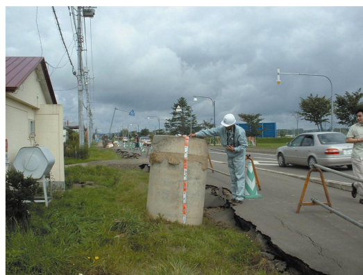
Photo 3: Risen manhole in Onbetsu City
