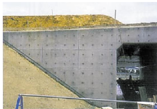
Photo 2: Box culvert after the repair
