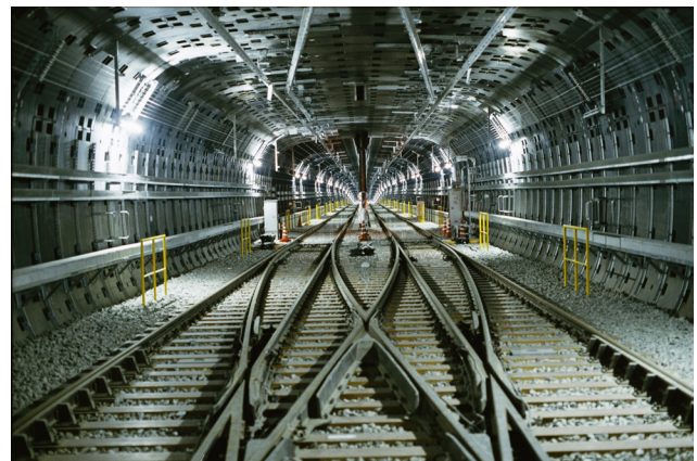
Photo 5: Completed crossover section (March, 2004)
