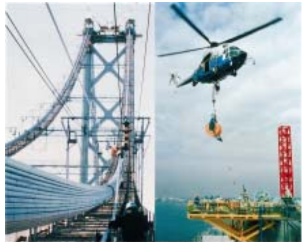
Photo 7: Cable strand construction (left), sea crossing of pilot rope (right) (Akashi Kaikyo Bridge)
