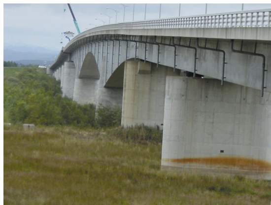
Photo 6: Torsion of the bridge axis toward the left bank (Tokachi Kakou Bridge)
