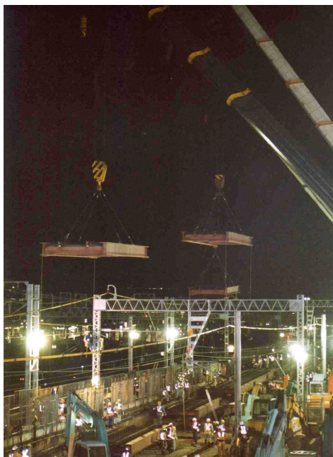
Photo2. Re-routings (withdrawal of temporary steel girders)
