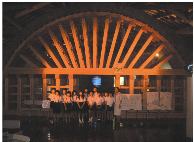
Photo 2: Full-sized wooden arch support
