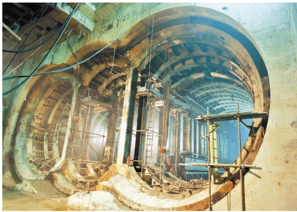
Photo 3: Shield machine steel shell
