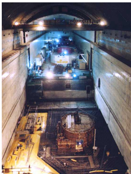
Photo 3 Expansion of the Existing Underground Power Plant
