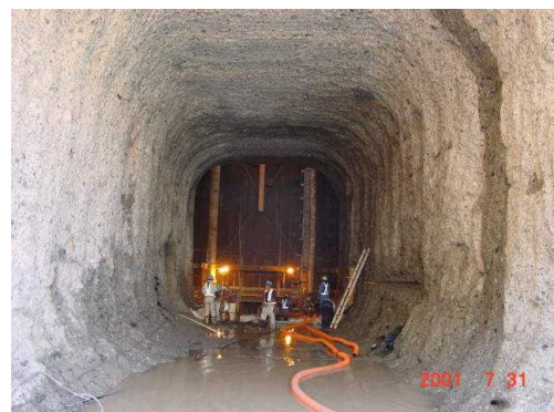
Photo 2 Boring of the Dam Body
