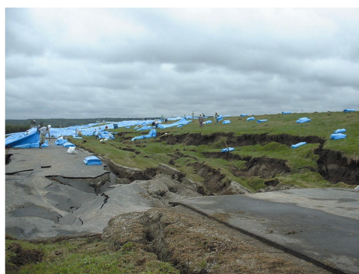
Photo 5: Damages to the embankment near the mouth of Tokachi River
