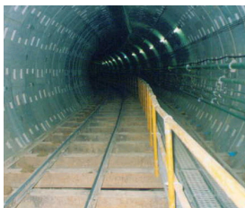
Use of segments with through bolts
