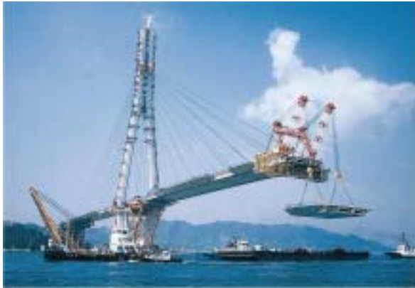
Photo 11: Overhang construction of the girder (Tatara Bridge)
