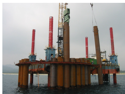
Photo-2: Driving work of bearing piles with use of 43m follower
