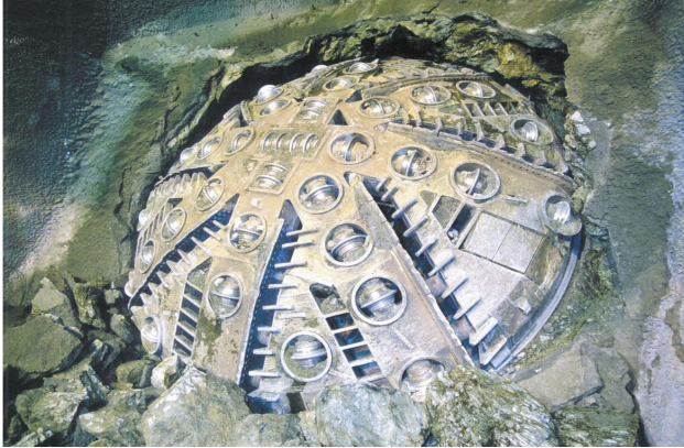
Photo 1: TBM reaching the inclined shaft
