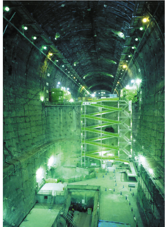
Photo 3: Underground power plant after excavation
