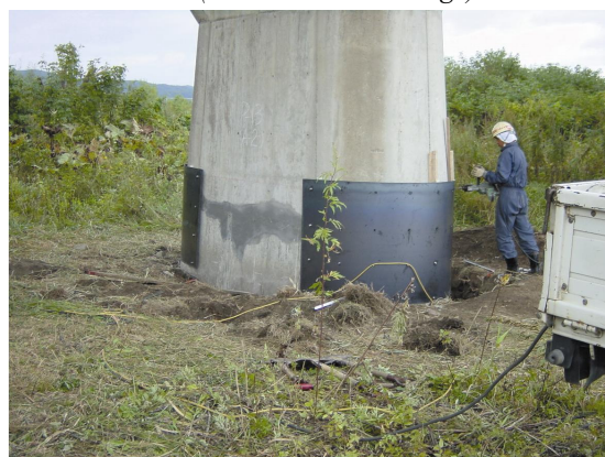
Photo 7: Steel Sheet adhesion reinforcement on the Chiyoda Ohashi
