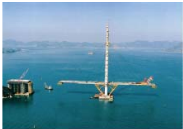
Photo 10: Balancing construction of the girder (Tatara Bridge)
