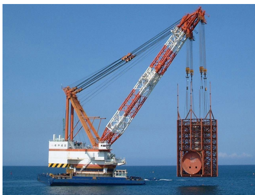
Photo-3: J-pipe installation work by a 1,600t hanging power floating crane
