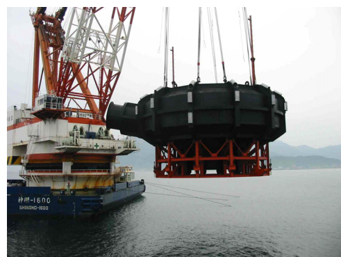
Photo-4: Installation of the multi-nozzle discharge
