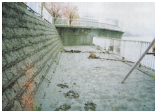
Photo 4. Damaged revetment and volcanic ash deposit at the hot spring resort on Lake Toya
