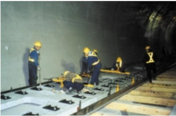
Photo 3. Laying track slabs; teamwork is the key
