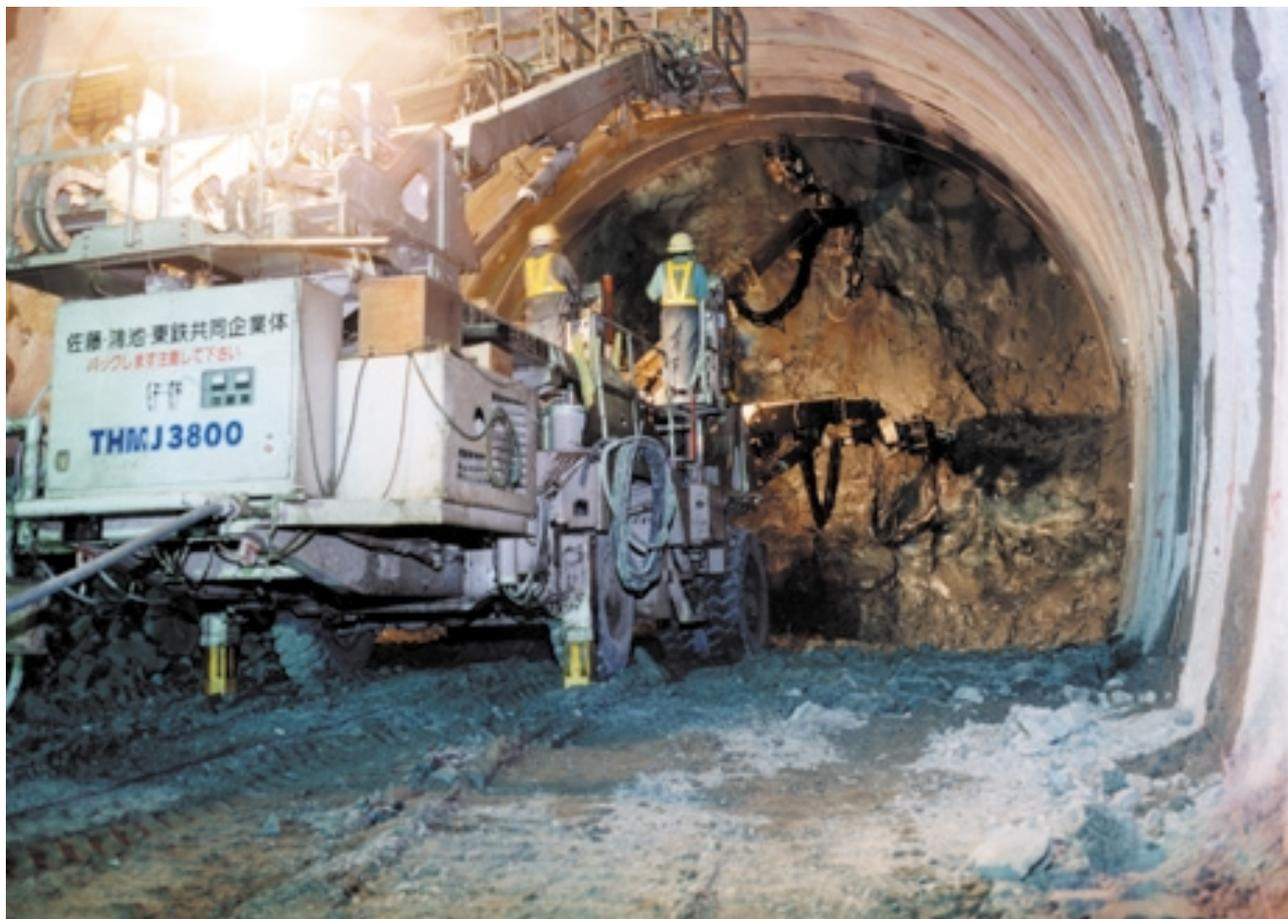
Photo 1. Blasting and excavating in the Torigoe construction section; efficient working in a complex geology
