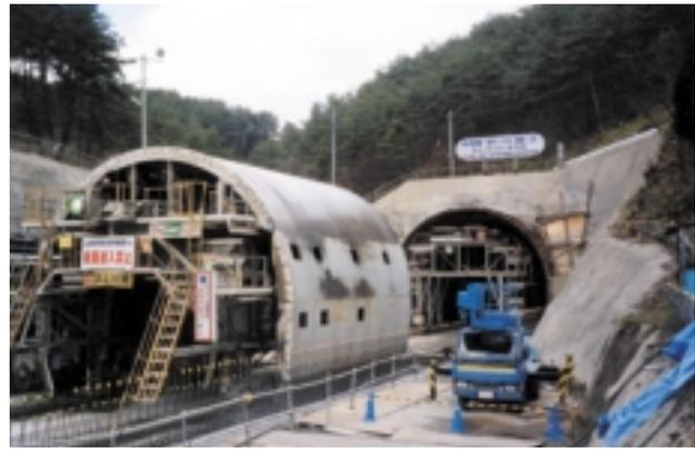
Photo 2. Movable form placed at the Tokyo portal of the Midou section
