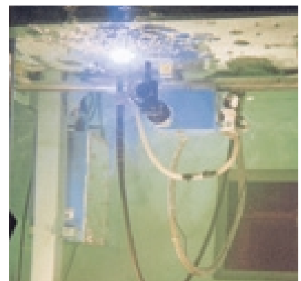
Photo 3 Underwater welding machine during experiment in overhead position
