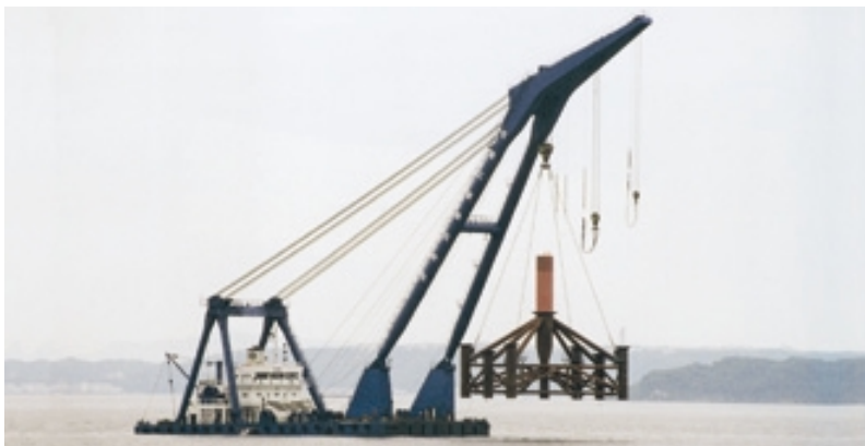
Photo 1 Steel jacket of mono-pod fender-type mooring dolphin
