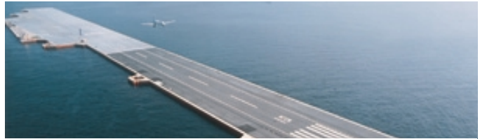
Photo 5 Low-approach flight tests to check proper functioning of instrument landing system on floating airport model
