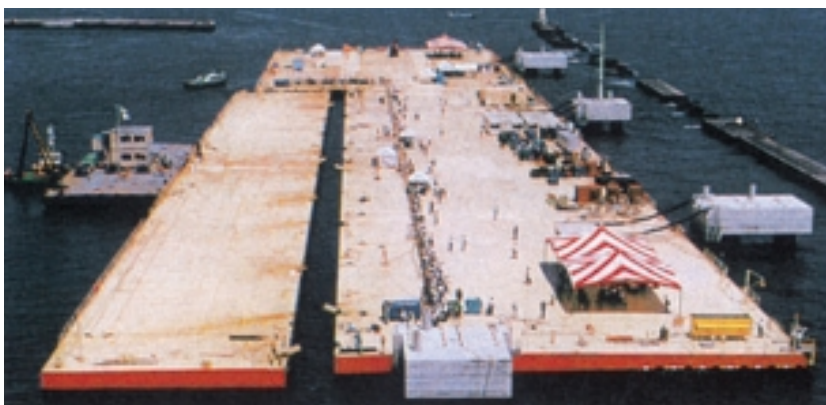
Photo 2 Public demonstration of joining operations in July 1996
