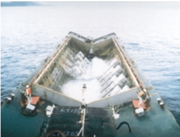
Photo 3 Blocks being dropped from open-bottomed hopper barge accurately located using DPGS
