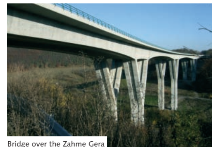
Bridge over the Zahme Gera
