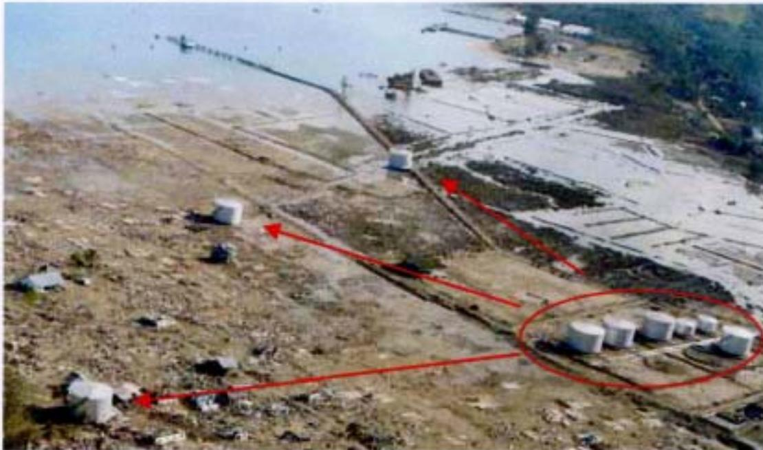
Figure 9.2 Displaced oil tanks by the tsunami
