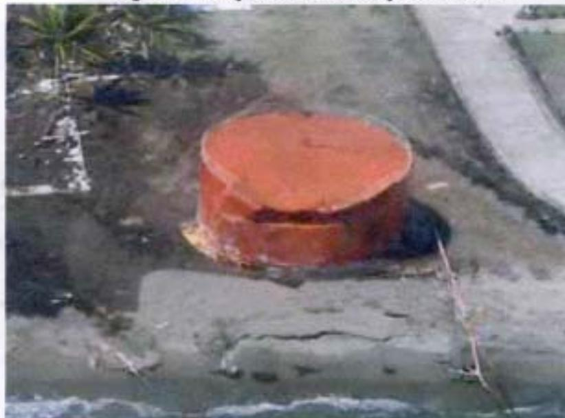
Figure 9.3 Buckled and settled tank at Meulaboh
