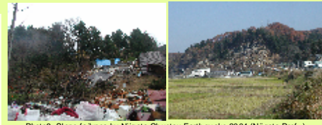
Photo3 Slope failures by Niigata Chuetsu Earthquake 2004 (Niigata Pref.)
