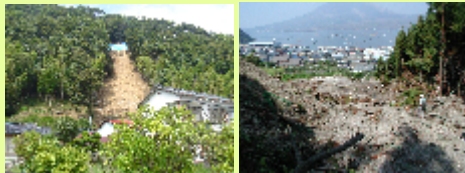
Photo2 Landslides caused by typhoon (2004, 2005)
