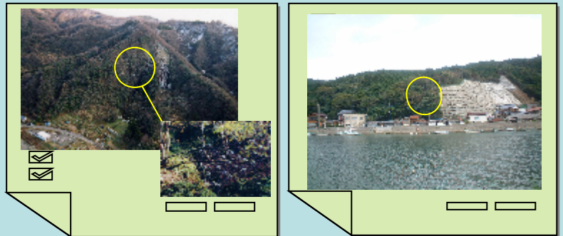
Non-frame in combining with concrete structures to protect natural slopes
