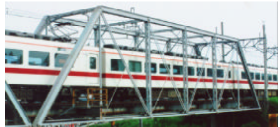
移設を待つ大谷川橋梁
