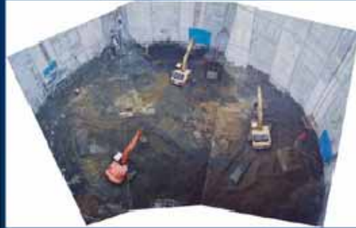
Excavation inside the Slurry Wall
