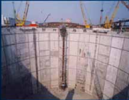
Overall View inside the Slurry Wall
