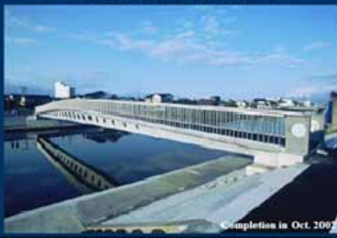
Completion of Sakata-Mirai Bridge
