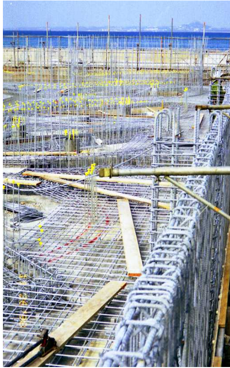
Galvanized Steel Rebar in Real Construction Site
