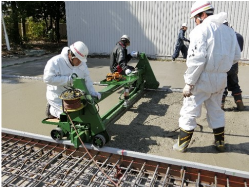
Photo F Simple finishing machine prototype ensures flatness
