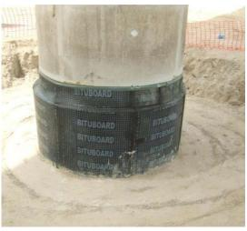
entering the concrete. In addition, the concrete itself was designed to be highly durable, consisting of low w/c ratio OPC and a blended mix to achieve low permeability. Simultaneously, this mix results in a 50% reduction in  $CO_2$  emissions.
