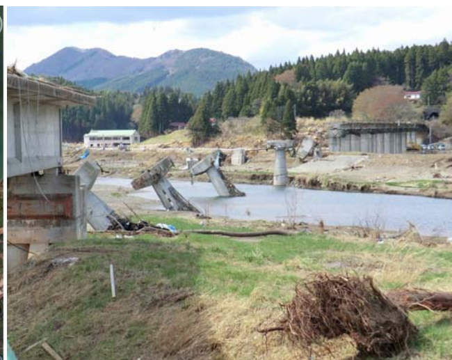
Fig.3 Inclined piers (Tsutanigawa bridge)
