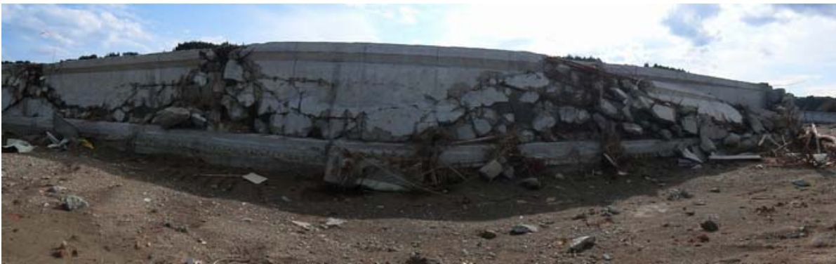
Fig.5 PC girder (Tsutanigawa bridge) washed away and damaged by tsunami
