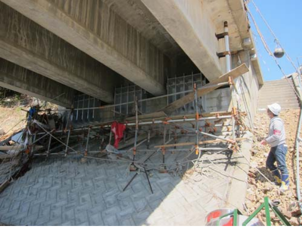
Fig.7 Device to prevent falling down of girders
