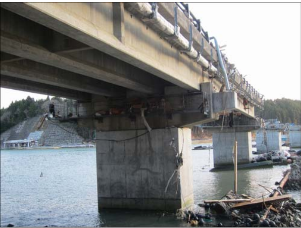
Fig.8 Seismic strengthening of piers (Utatsu-ohashi bridge)
