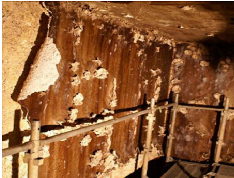
Photograph-2 Detachment of coating-type lining
