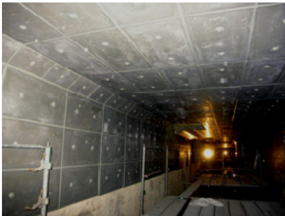
Photograph-5 Walls and ceiling in inflow channel
