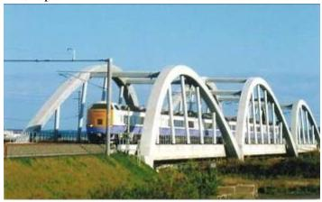
seismic lateral reaction force of the bridge deck suspended from the arch ribs can be resisted at the abutment. In order to realize this structure, new devices were developed such as large capacity reinforced concrete stoppers and suspenders absorbing deck shrinkage due to creep and drying shrinkage of concrete.
