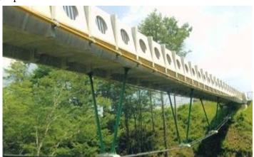
adopted. The primary and secondary cables were also used at the erection stage to support the deck self weight and adjust the deck sag, respectively. A solid handrail takes into account the structural system, and the U-shaped deck heightens the bending stiffness and reduces pedestrian vibration.
