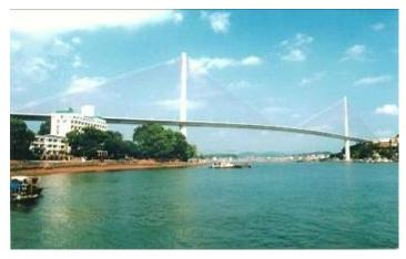
cross-section deck reinforced by steel column braces. A prestressed concrete structure was also adopted at the lower part of the towers so as to increase the resiliency. The bridge reveals the advanced bridge engineering technology of Japan and the Japanese latest technology was transferred to the Vietnamese engineers.
