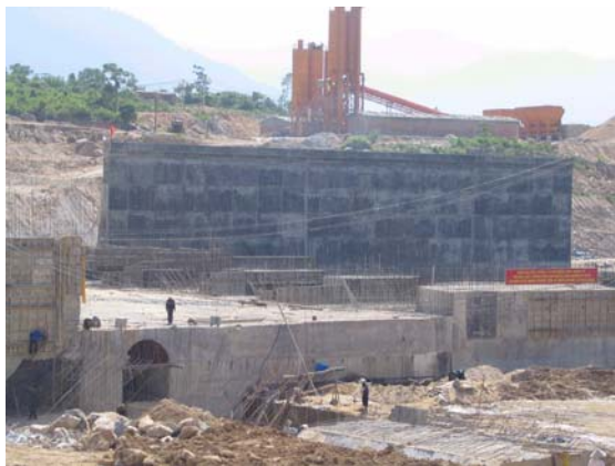
Photo 1 RCC at Dam PlayKrong (Kontum Province, Vietnam)
