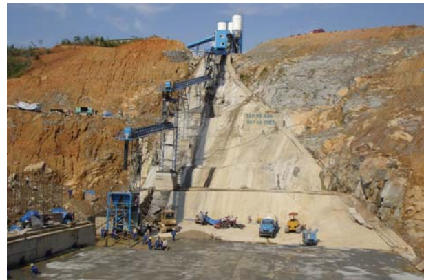
Photo 2 RCC at Dam Dinh Binh (Binh Dinh Province, Vietnam)
