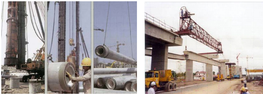
Photo 2 High performance concrete applied in construction at Viet Nam
