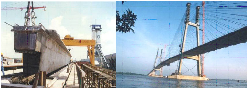
Photo 1: Viet Nam My Thuan bridge was built by high performance concrete
