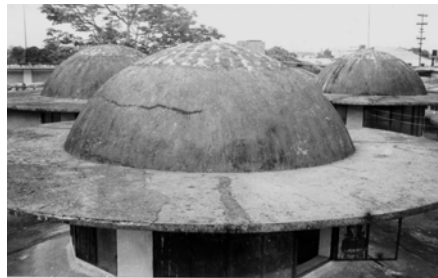
Figure 7 Cracks in concrete structures situated under action of HHC
