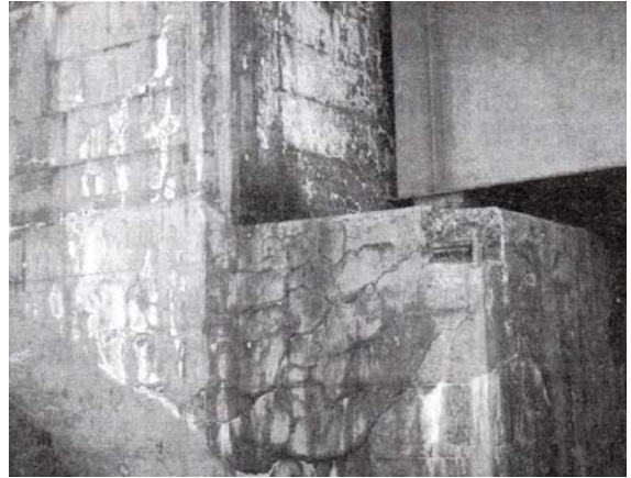
Photo 1 Damage due to alkali-aggregate
