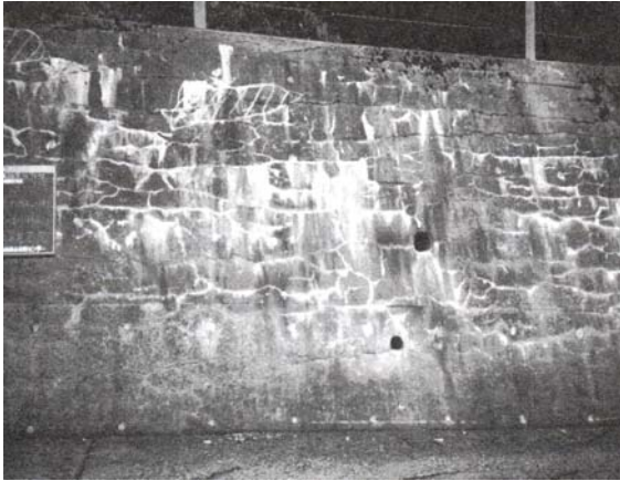
Photo 1 Damage due to alkali-aggregate
