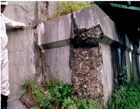
Photo 2 Frost damage
