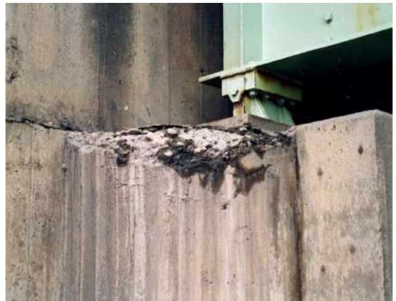
Photo 2 Frost damage
