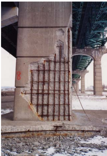
Photo 3 Corrosion of reinforcing bars
