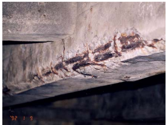
Photo 3 Corrosion of reinforcing bars
